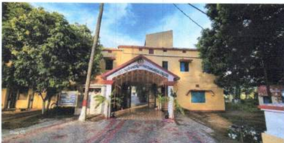
Administrative Building Gate
